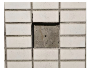
2) Wall Surface after Tile Removal
